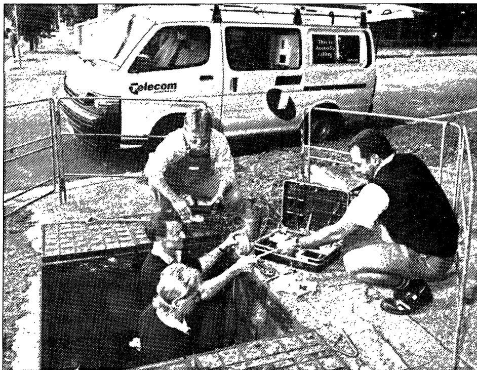
Laying cable in Centennial Park
