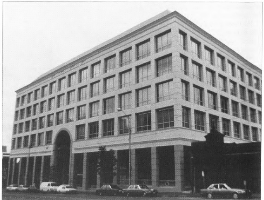
The new Southern Command H.Q. (Pictures by Keith Livingston)
