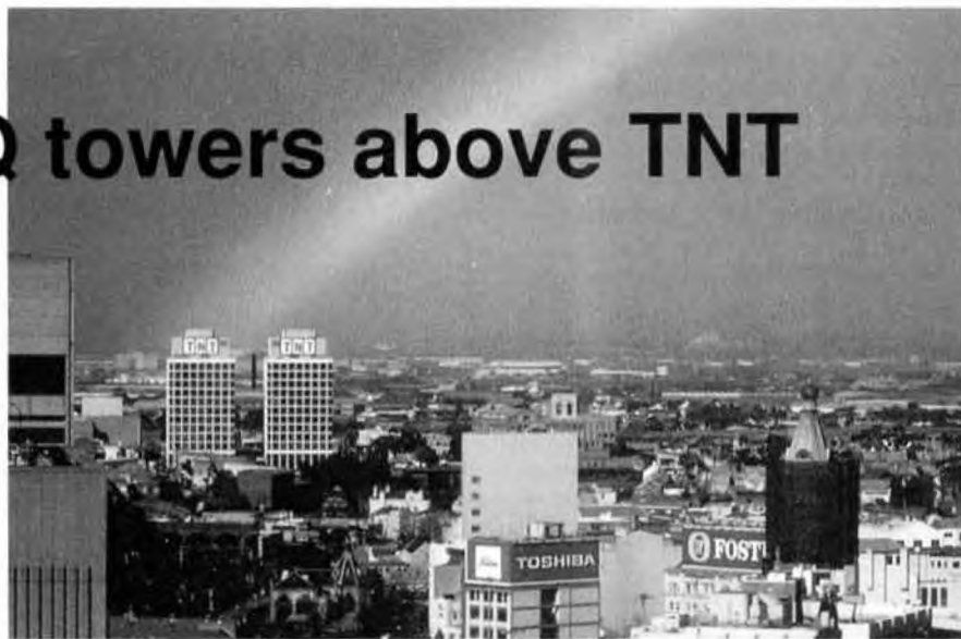
Impressive from a distance, TNT Tower No.2 gave no indication of the well-worn interior when occupied by the AFP.
