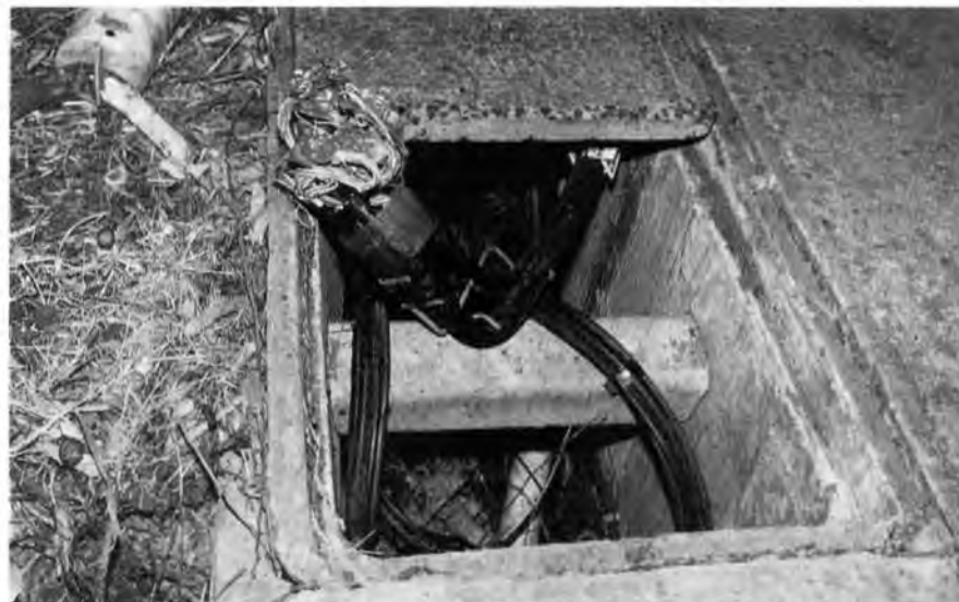
Damage to telephone lines caused by a suspect attempting to physically intercept a telephone line for the purpose of gaining free and untraceable communication links with an overseas computer system. The suspect was arrested before he could achieve his objective.
