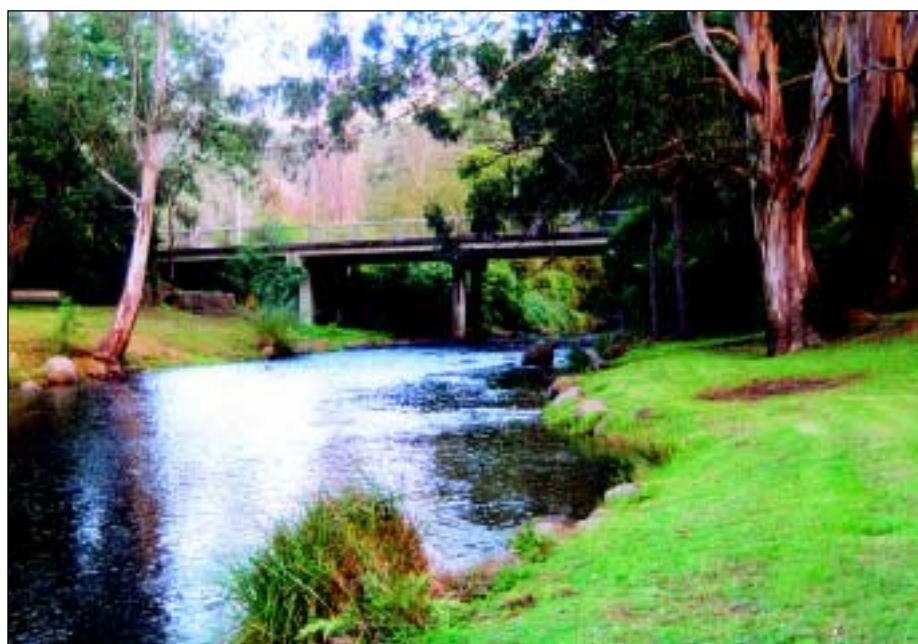
Figure 3: The Blackwood Avenue landslide lies on the north bank of the Yarra River at Warburton. The toe of the landslide is at the edge of the river. In the unlikely event of a total blockage of the river, infrastructure such as the bridge spanning the Yarra River could be affected.
