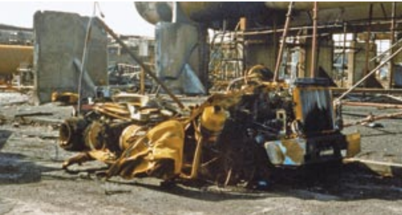
Field skills for students involve working in arduous conditions and real-life situations
