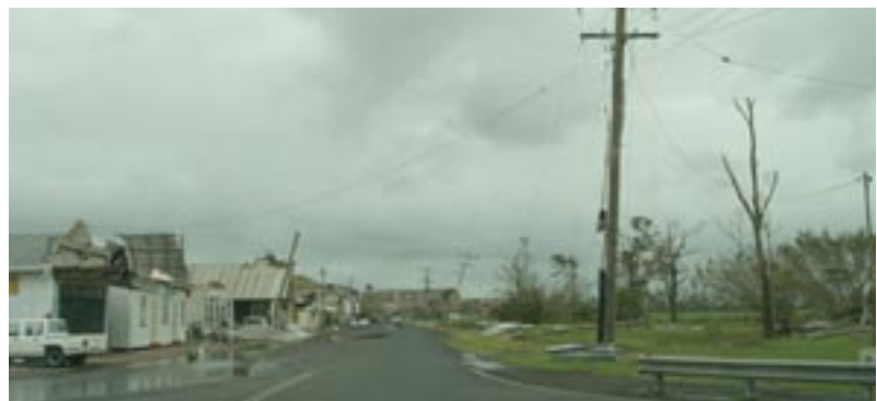
Cyclone Larry destroys buildings and vegetation and floods the local area.
