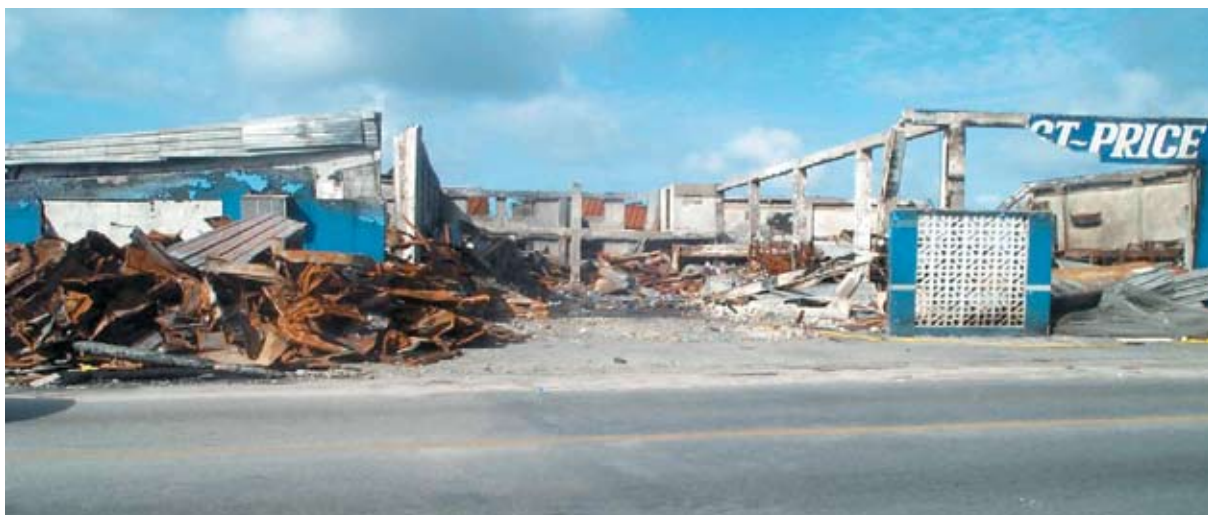
A major structure fire in the Marshall Islands in 2005 had a severe impact on the national economy.
