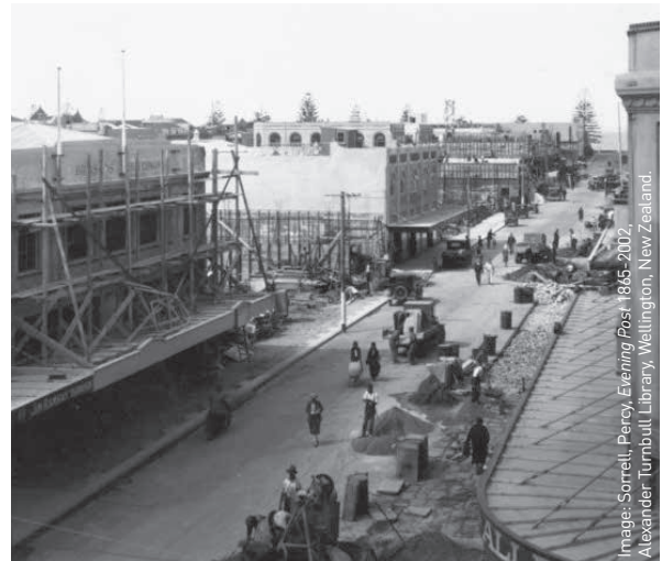
Men working on the road and buildings in Emerson Street, Napier, after the earthquake of 1931.
