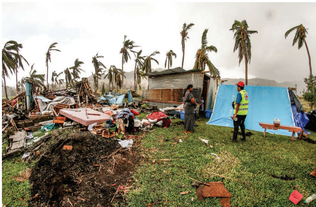
Cyclone Winston destroyed or damaged more than 32,000 homes on its path through Fiji in February 2016. Image: IFRC, Navneet Narayan.
