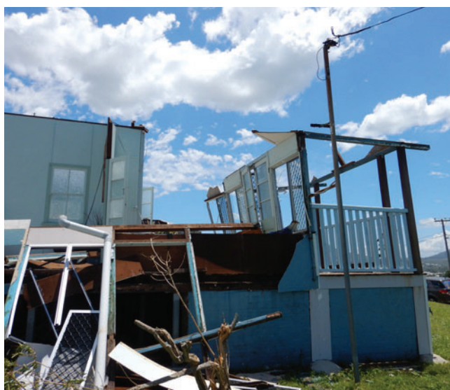
Tropical Cyclone Marcia caused significant damage to property in Yeppoon, Queensland due to its severe winds.
