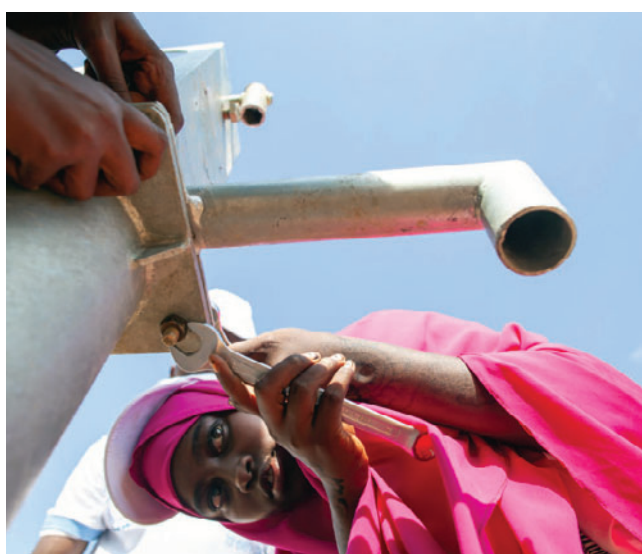
Muslima, age 18, from Somalia learns how to install a water pump at a centre that provides training to displaced youth in construction, engineering and plumbing.
