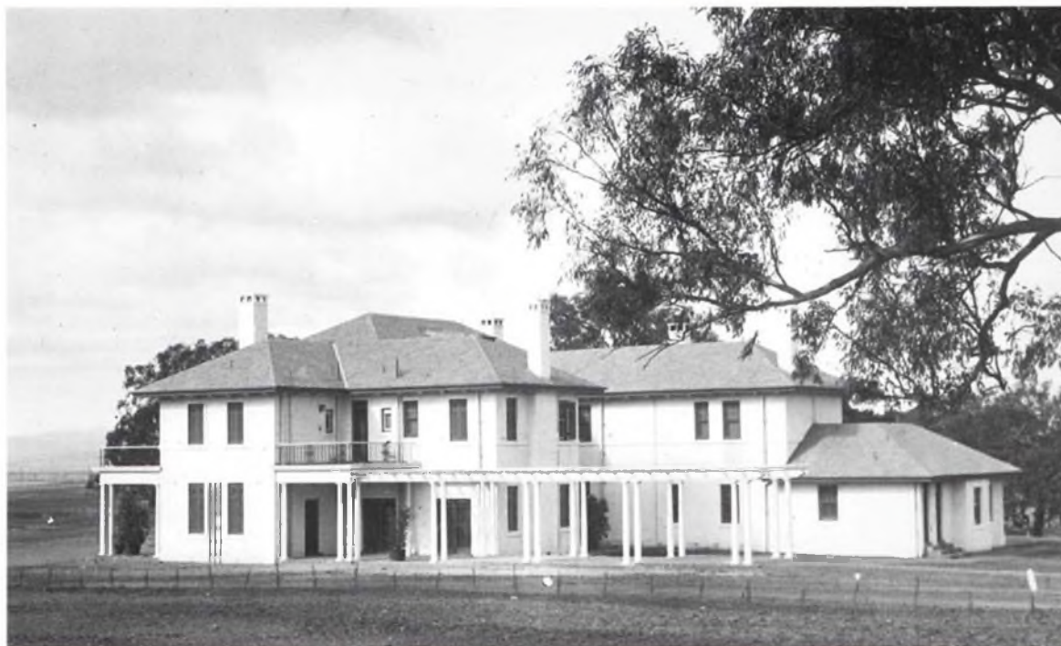
The completed Prime Minister's Lodge, 1927. Photo: W J Mildenhall. NLA 26520. Reproduced by permission of the National Library of Australia.
