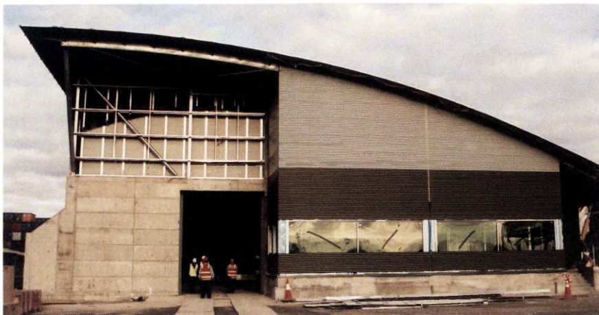
The container x-ray scanning hall stands 12.5m high and is 43m deep: in Melbourne the facilities have been built on silt so 25m pylons were sunk into the ground to stabilise the structure.
