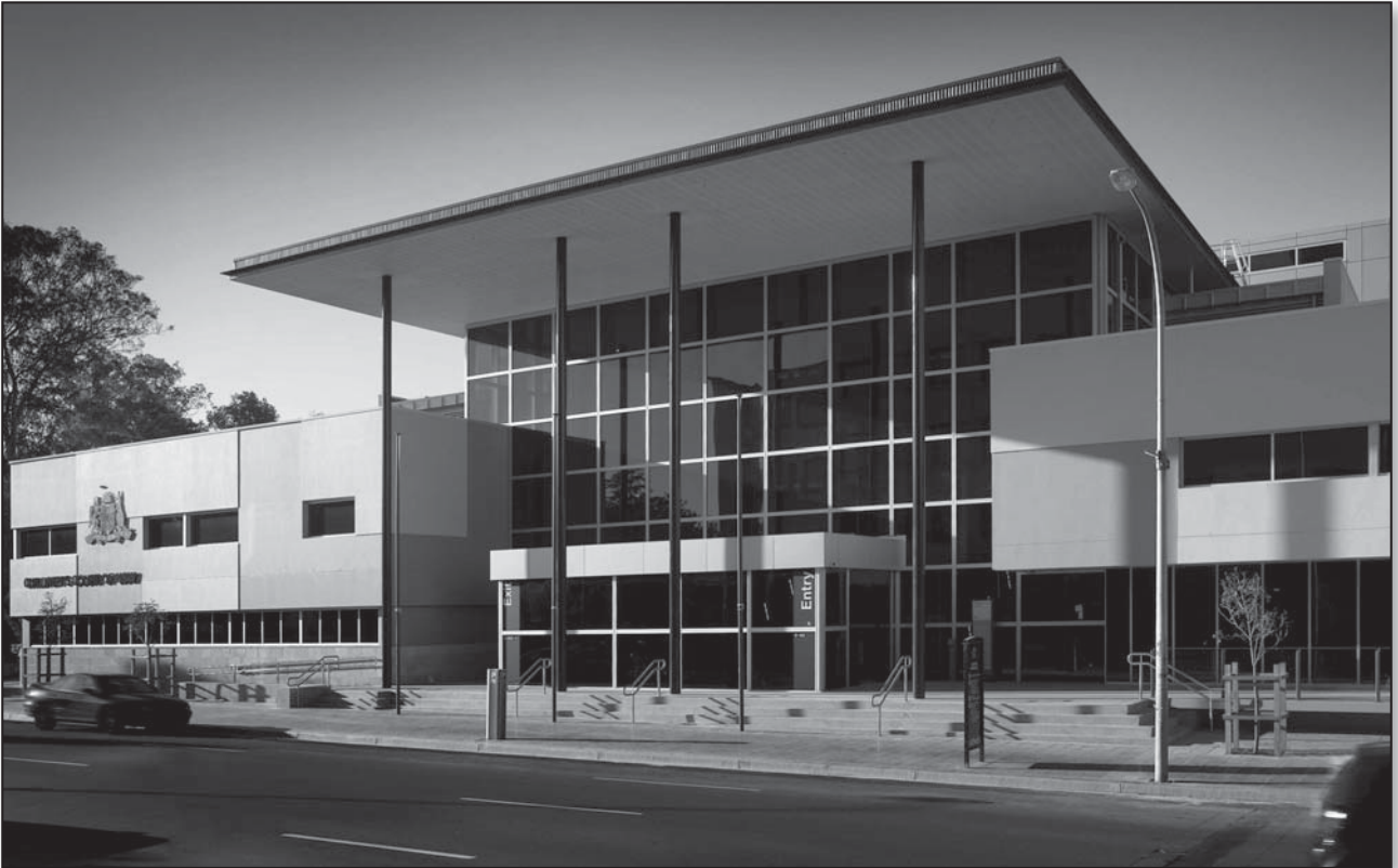
The Sydney West Trial Court Complex.
