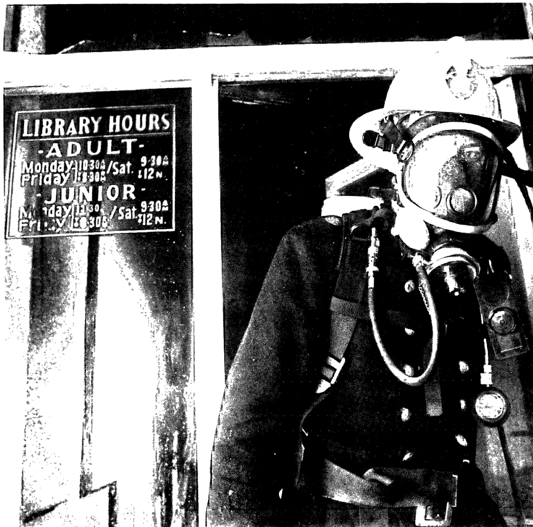
Above: Gas-masked firefighter emerges from the charred shell of the Maroubra Library. Noxious fumes delayed the efforts of staff to begin the massive clean-up. Once inside the library staff were aghast at the scale of damage — as well as fire and water damage a thick layer of black carbon soot covered books, shelves and furniture. Police suspect vandals may have entered the building on a Saturday after the staff had left at noon. It looks as though material from around the circulation desk (transaction cards, books awaiting processing etc) was piled up and lit. The material smouldered overnight. Heat built up blowing out windows allowing oxygen to fuel the fire to a blaze. This alerted local residents. The fire brigade broke in to fight the fire on Sunday afternoon.
