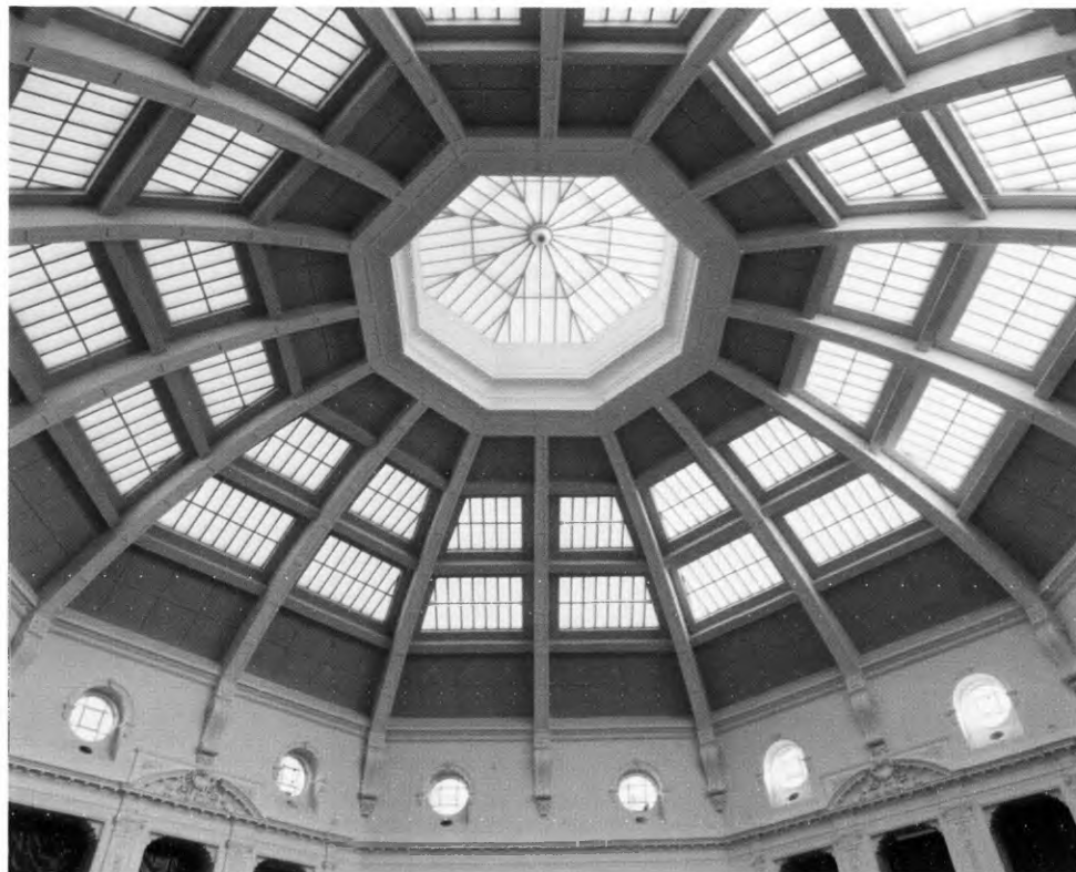
Looking up to the refurbished dome
